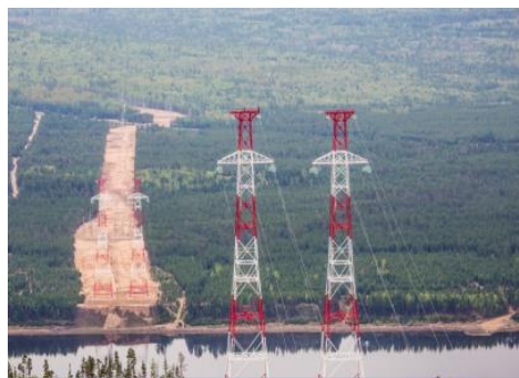
Trunk line underwater crossing over the Angara river, AT-105
