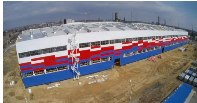
«Russian Electric Motors» plant, Construction metal structures
